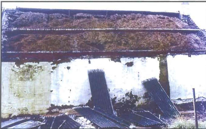
The removal of a zinc roof exposes the long-forgotten thatch underneath at a cottage in Hook.
